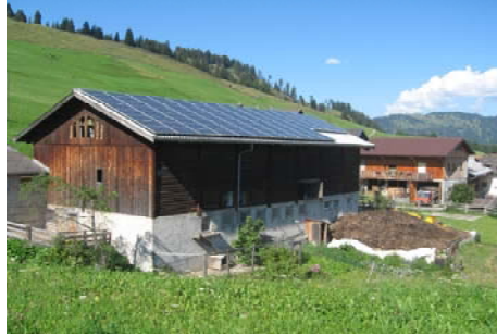
Photovoltaikanlage Martin Simonett, Lohn
